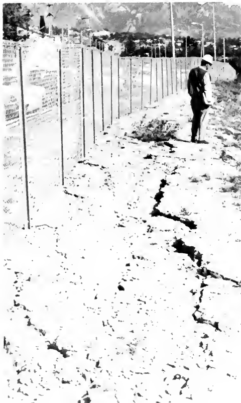
Photo 2. Cracking along top of cut slope on Route 210.
